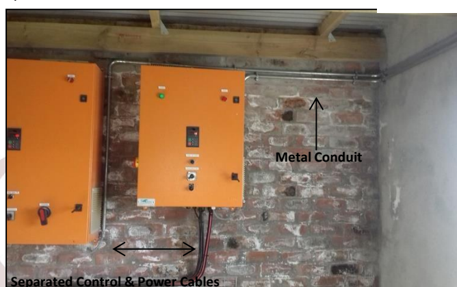
Figure 5- Control cable installed in metal conduit and high voltage cables separated from control cable
