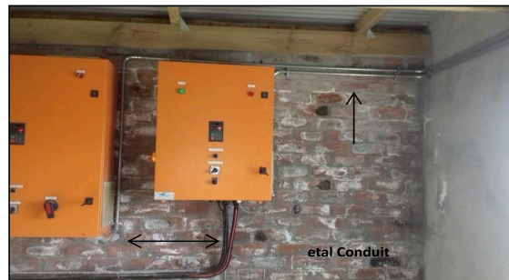
Separated Control & Power Cables
